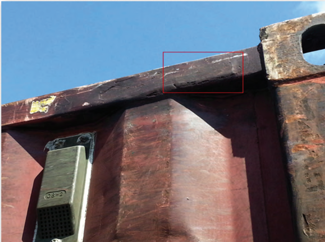
Container Inspections Should Detect Altered Container Frames
